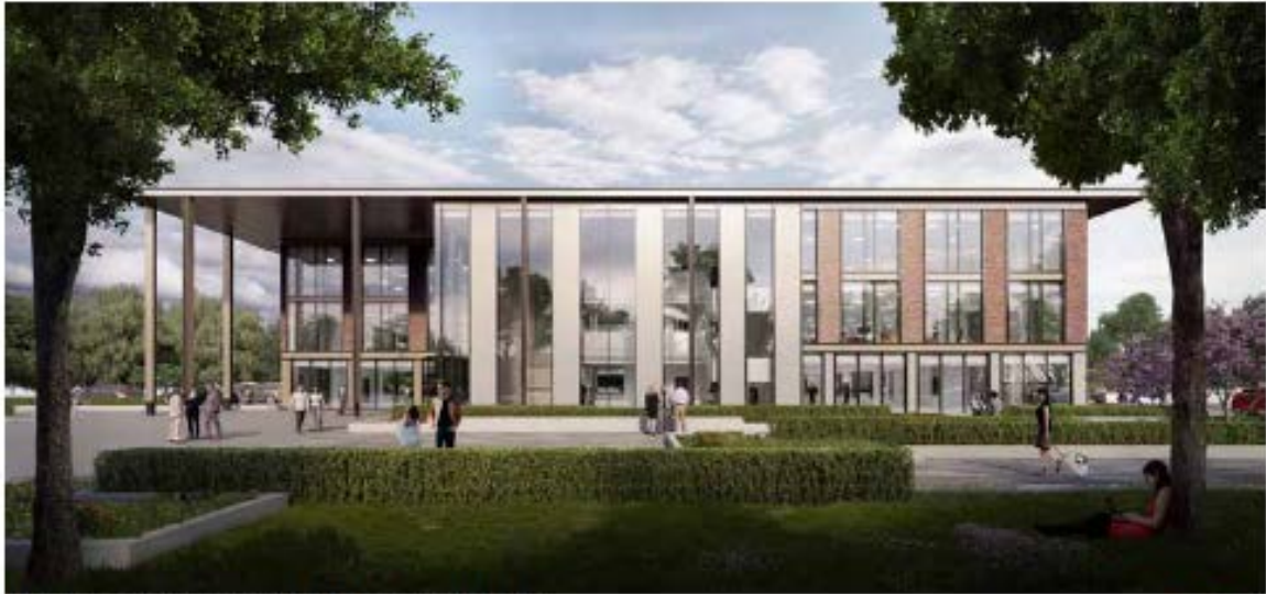
Building 1 Croxley Park - under construction
